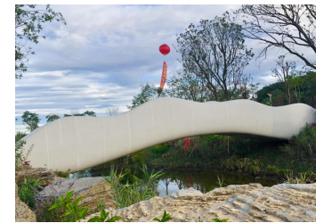
The Second 3D Printing 'Bridge Fujian Quanzhou 3D Printing Bridge' Completed
