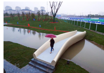
Shanghai Taopu 3D Printing Bridge Completed, which is Reported by National Documentary "MADE IN SHANGHAI"
